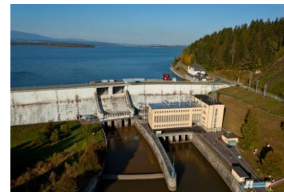
Orava hydro power plant
